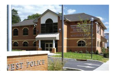
shaft). Combining wood and steel construction in walls and roof systems allowed for larger spans in the building and floors capable of supporting unusually heavy loads. Energy efficiency was embedded during modular construction and enhanced by final construction tasks undertaken at the site (e.g., special insulation board installed during the construction of the brick exterior).
